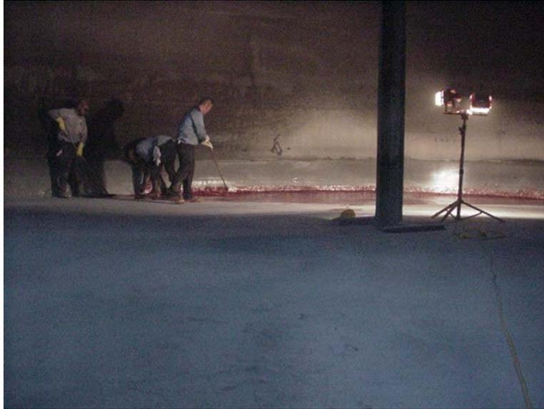
Figure 3: Steel Tank Lining, Chemical Resistant Topcoat
